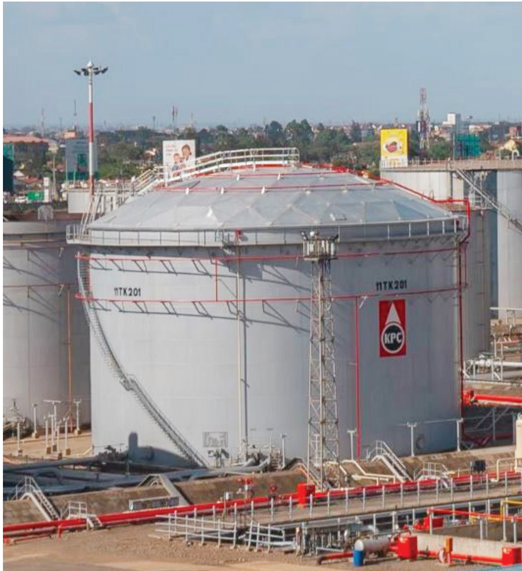
Sample sprit tank with dome roofing.
