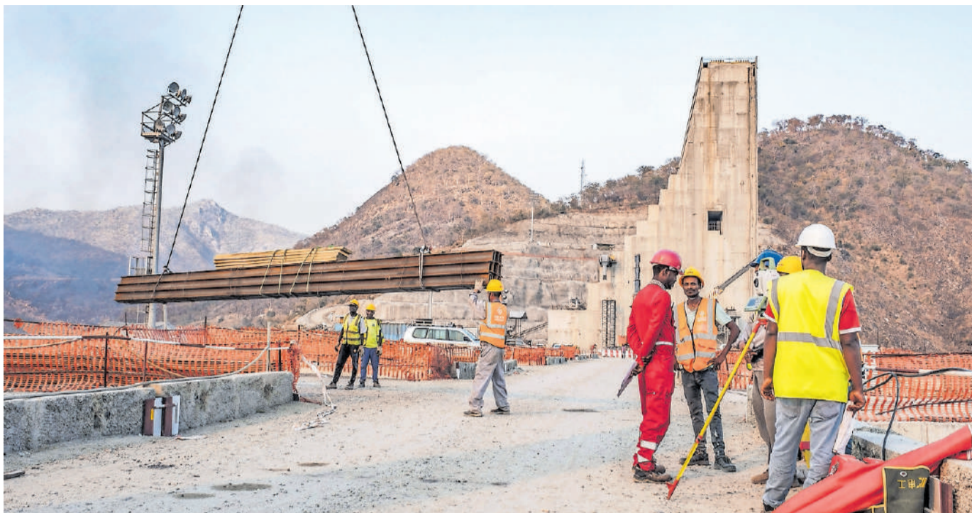
Construction works at the Grand Ethiopian Renaissance Dam near Guba in Ethiopia in December 2019. The dam, a 145m-high, 1.8km-long concrete colossus, is set to become the largest hydropower plant in Africa. Picture: AFP
