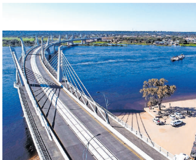
An aerial view of the newly built Kazungula bridge over the Zambezi River in Kazungula, Botswana. A new road and rail bridge linking Botswana and Zambia was inaugurated on May 10, 2021. Pic: AFP
